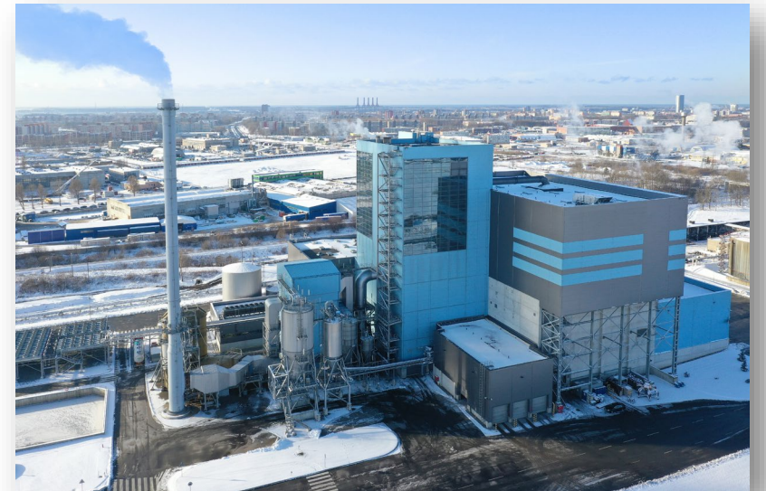
Gren WtE plant in Klaipėda, Lithuania
